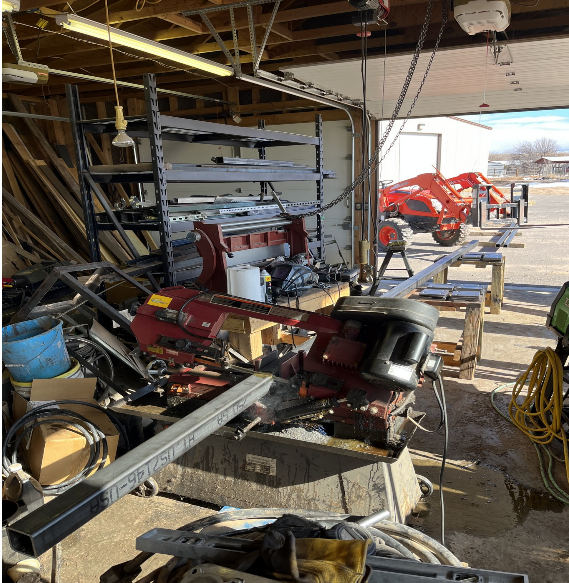
Figure 24. Cutting 40" long pieces of steel tube for the rail support posts.
