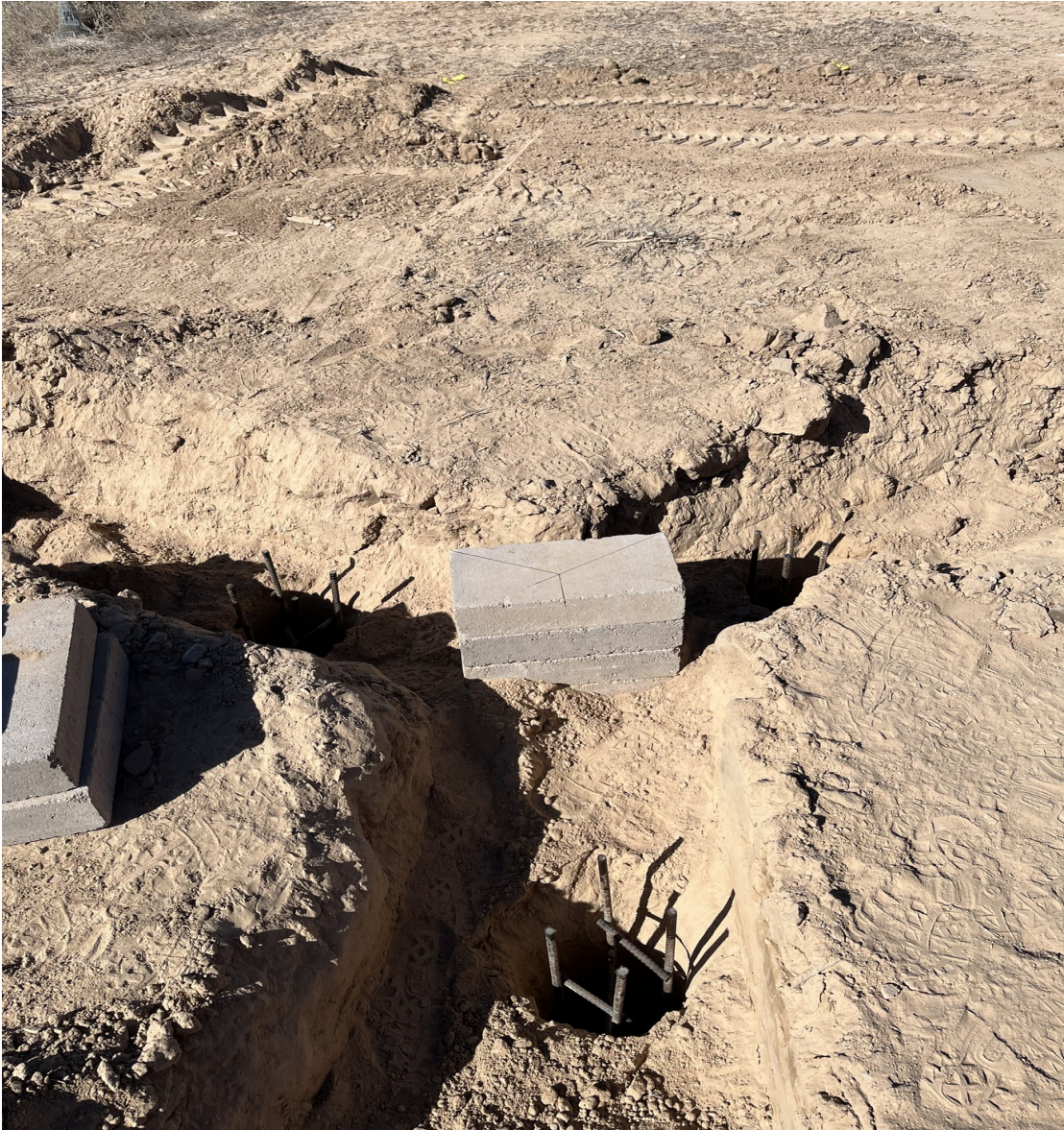
Figure 10. Rebar structures are in position in the pier holes.
