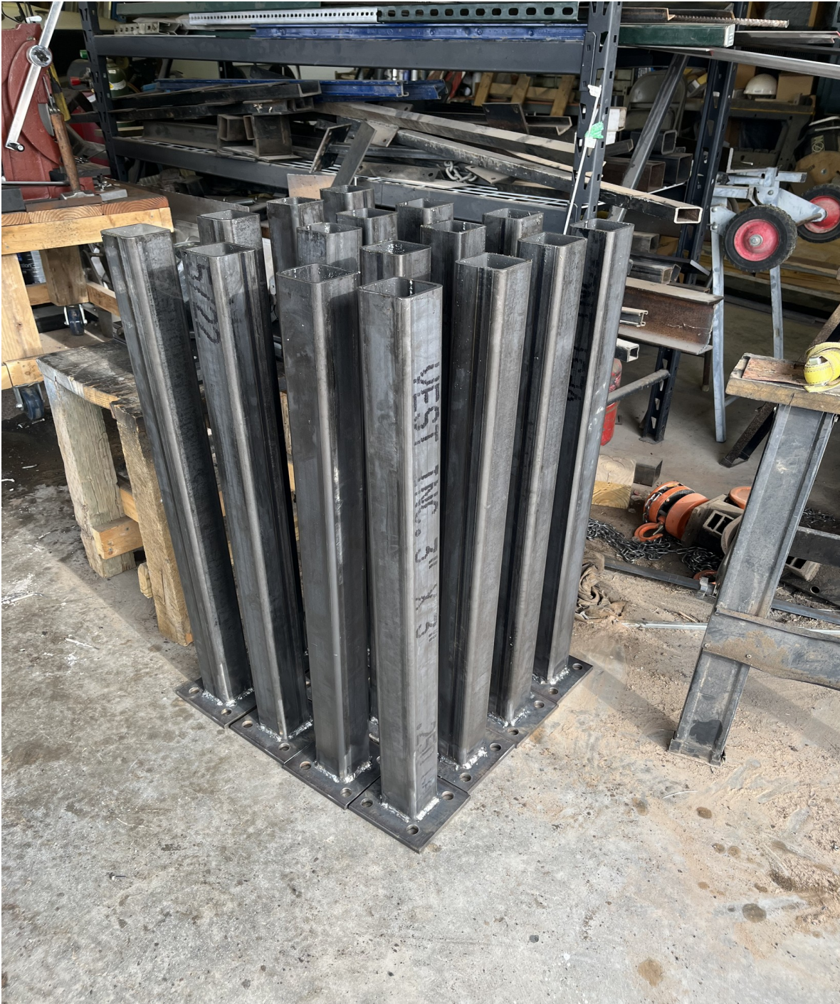
Figure 27. All 16 rail support posts have flange plates welded to them.
