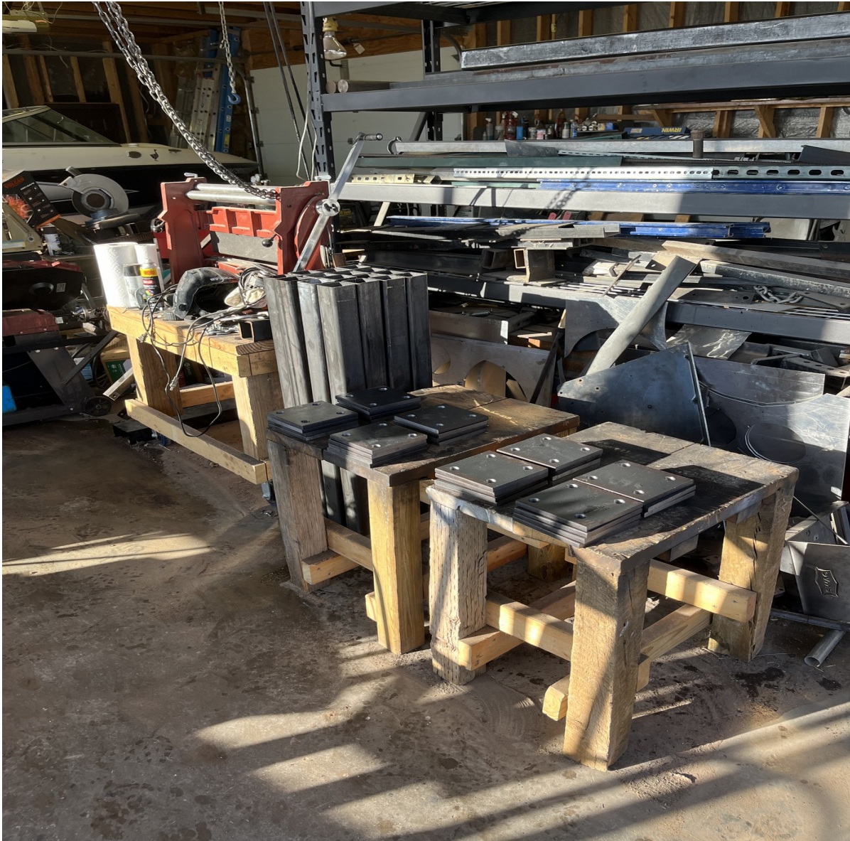
Figure 25. Rail support posts and support post flange plates are shown above ready to assemble the complete rail support posts (16FEB2023).
