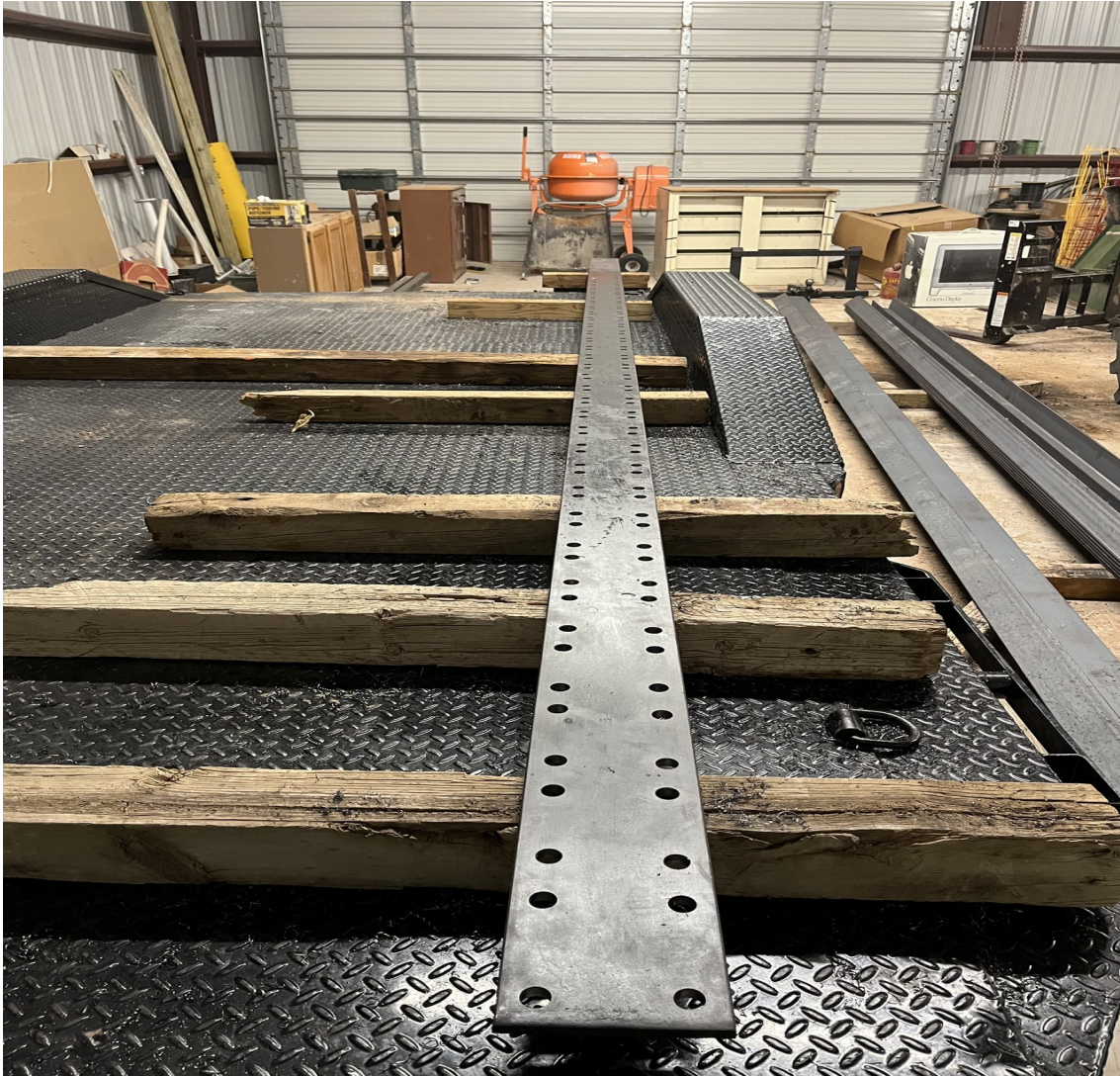
Figure 21. The 6"x1/2"x20' steel bar has been bored with 128 13/16" diameter holes (4 holes per 6"x6" plate) for the threaded rods that will be used to adjust the height of the circular rail (15FEB2023).
