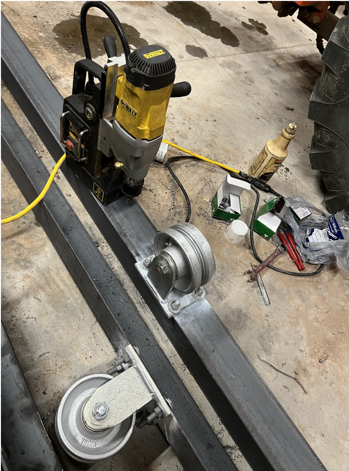
Figure 5. Two center side pieces with wheel assemblies bolted in place.
