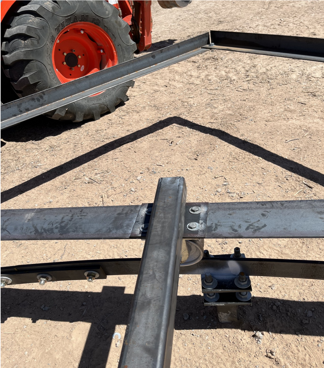
Figure 31. A flange for a truncated square side is bolted to the side piece with the spoke end in position to be welded onto the flange (7APR2023).
