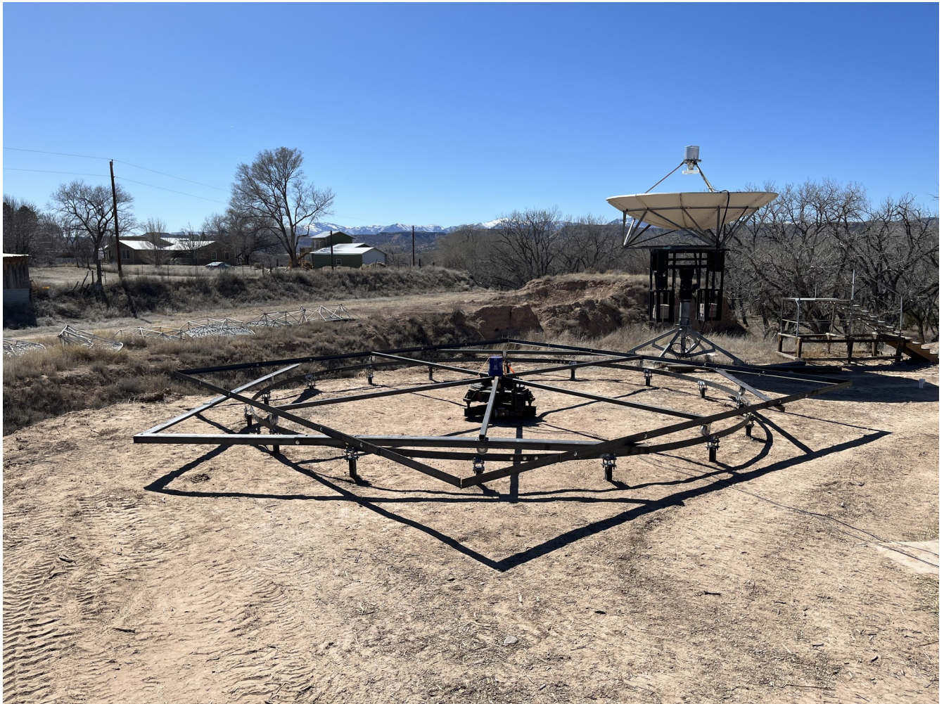
Figure 17. One corner of the truncated square base structure is completed.
