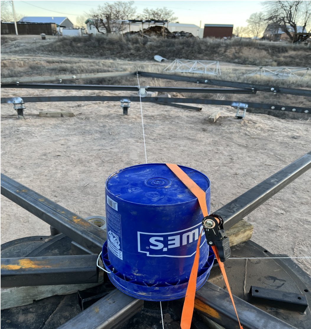
Figure 14. A corner-to-corner string across the full square base structure shows that the truncated square position for the ‘southwest’ wheel is not perfect.
