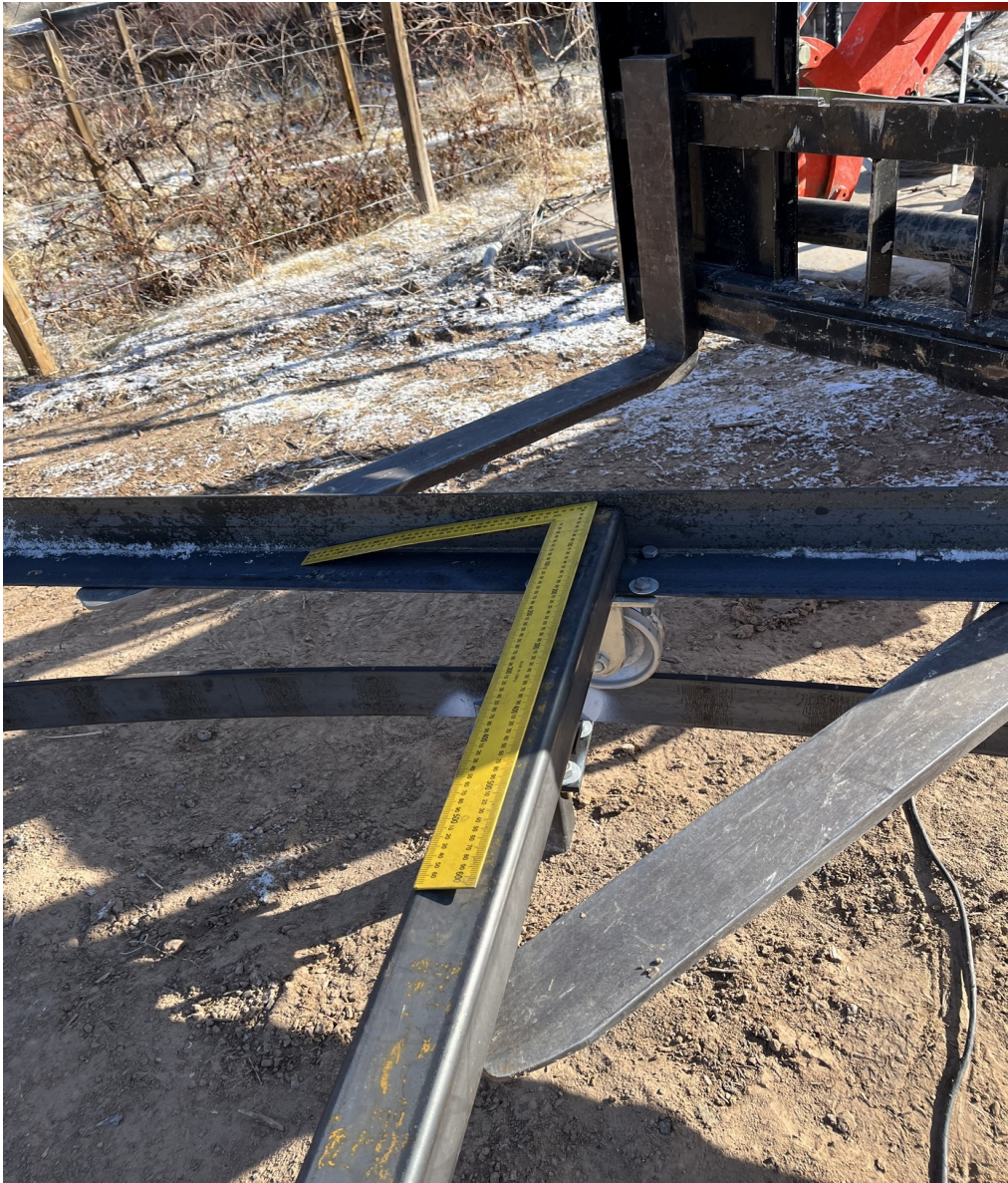
Figure 8. Using a carpenter's square to ensure things are square and true.
