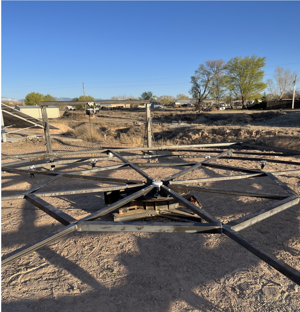
Figure 40. Spoke stiffener beams have been welded between adjacent spokes (16APR2023).
