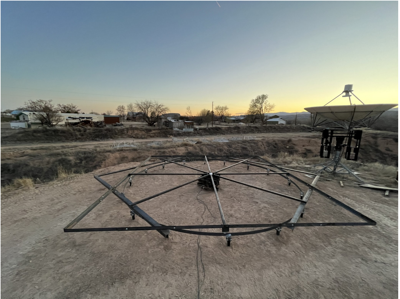
Figure 36. All spokes are installed and initial rotation testing has begun (11APR2023).
