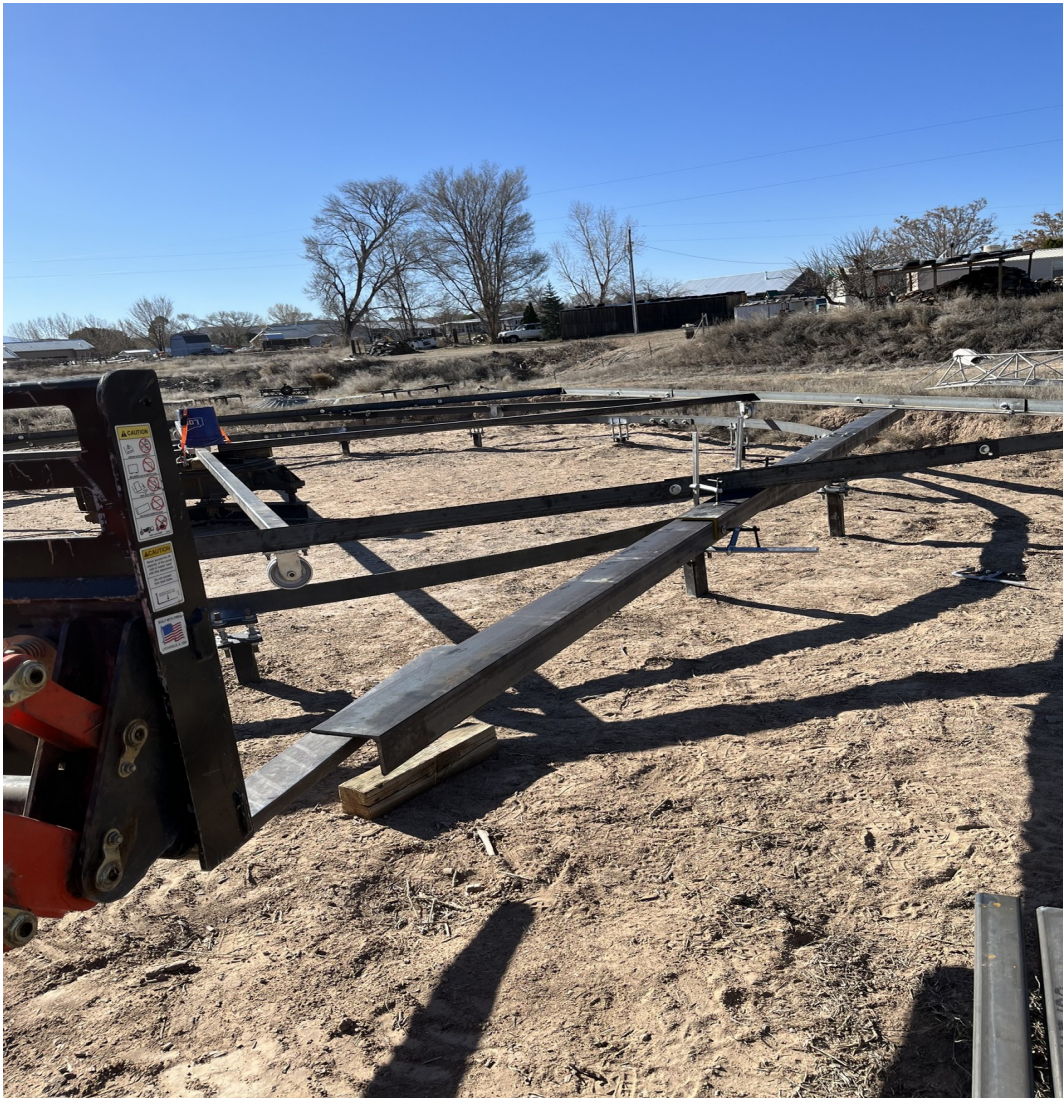
Figure 19. Using forks to assist in assembling the corner angle beams.
