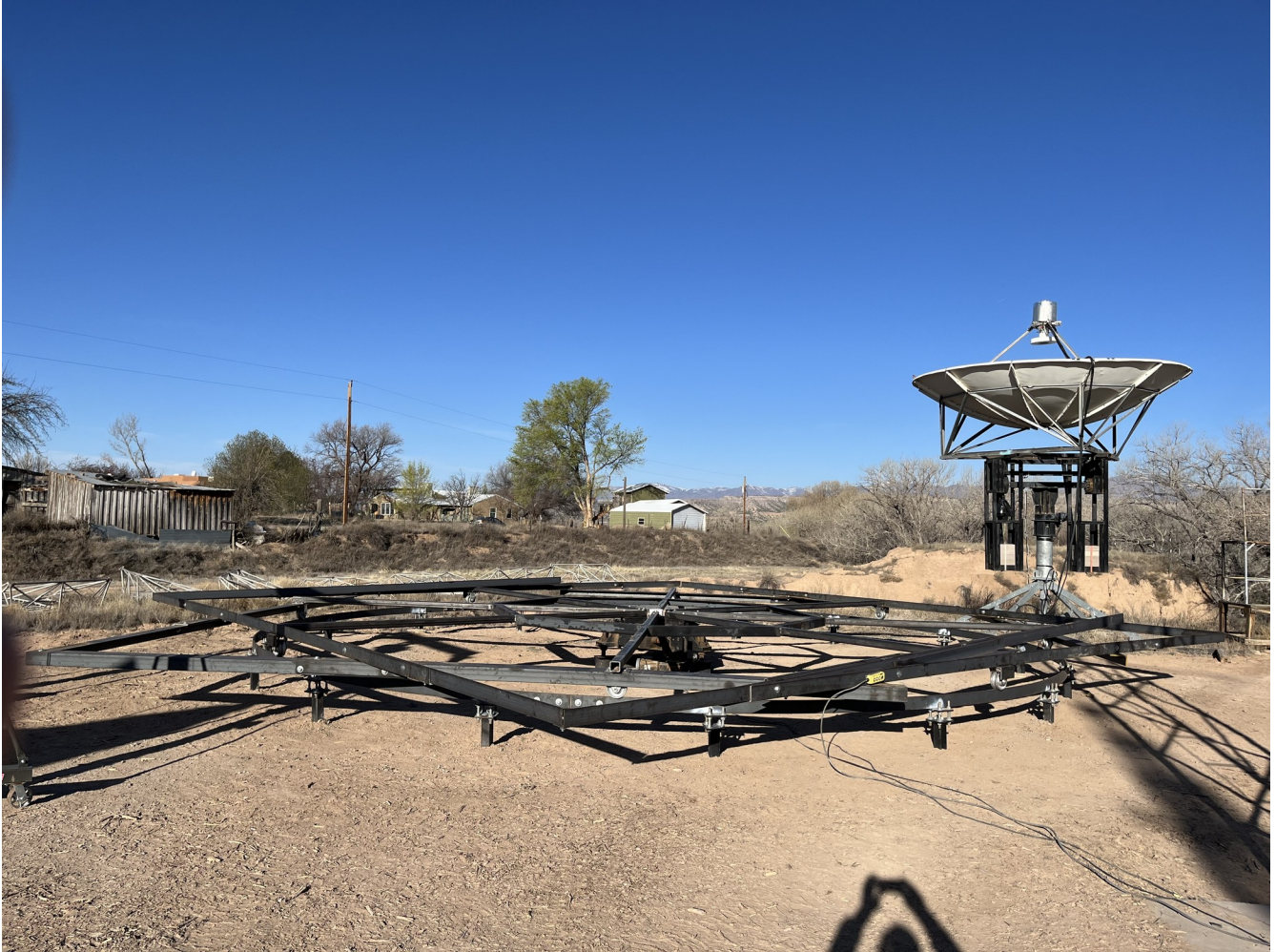
Figure 41. AZ rotation platform is fully assembled (17APR2023).
