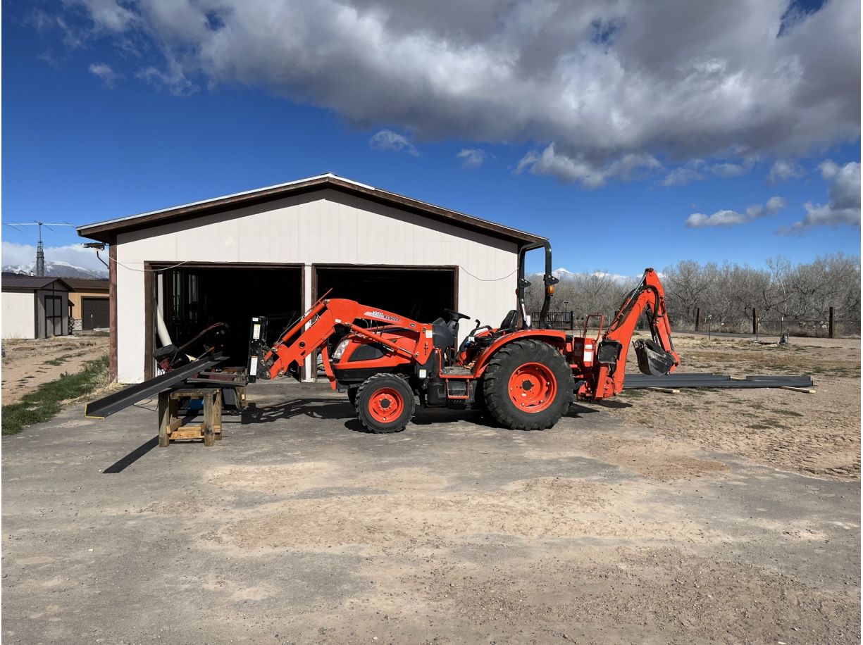
Figure 12. Using a tractor with forks to load the heavy beams into the metal saw (31MAR2023).
