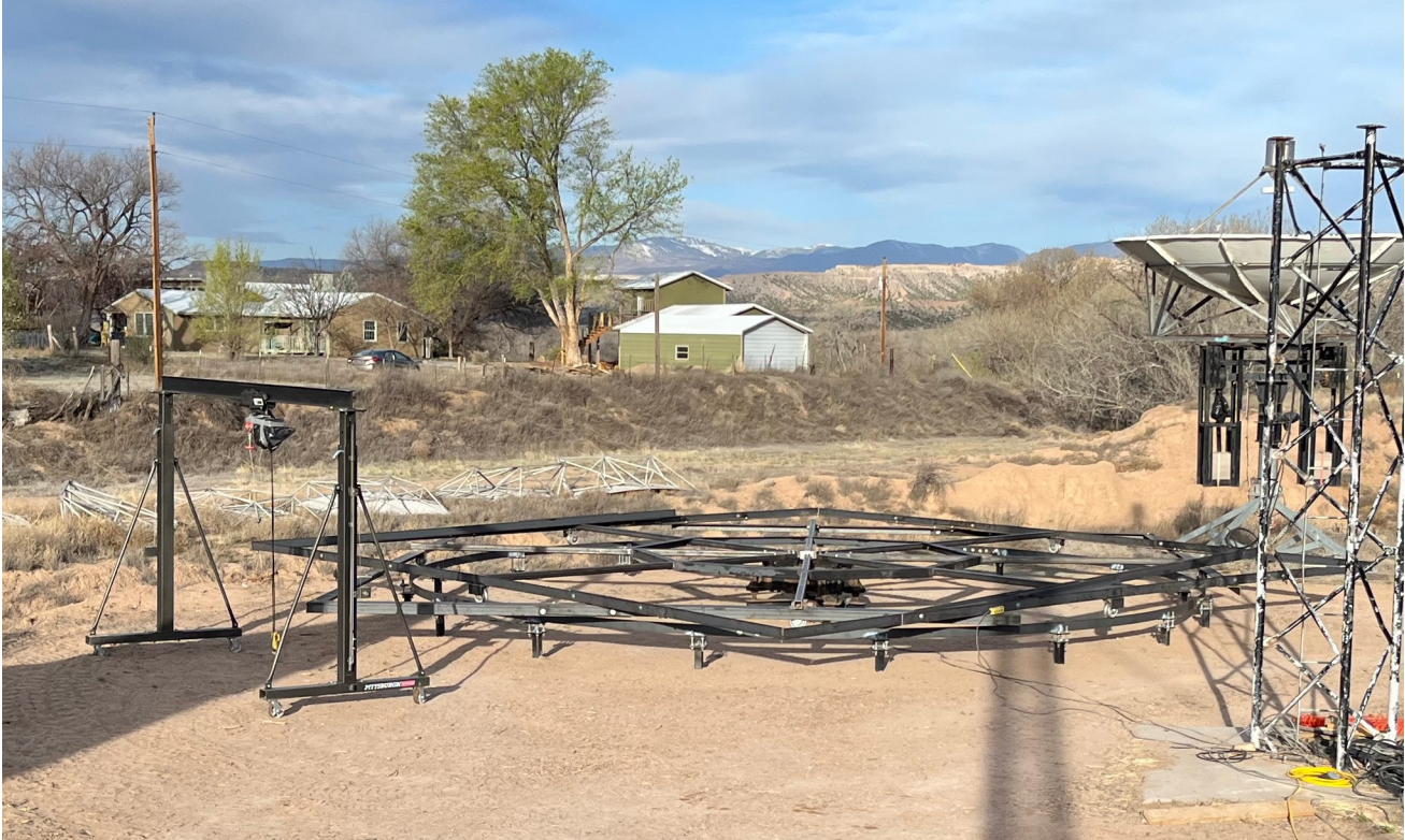
Figure 1. A portable gantry with electric steel-cable hoist is shown in approximate position to aid in assembling beams to form a lift tripod on the rotating structure (19APR2023).
