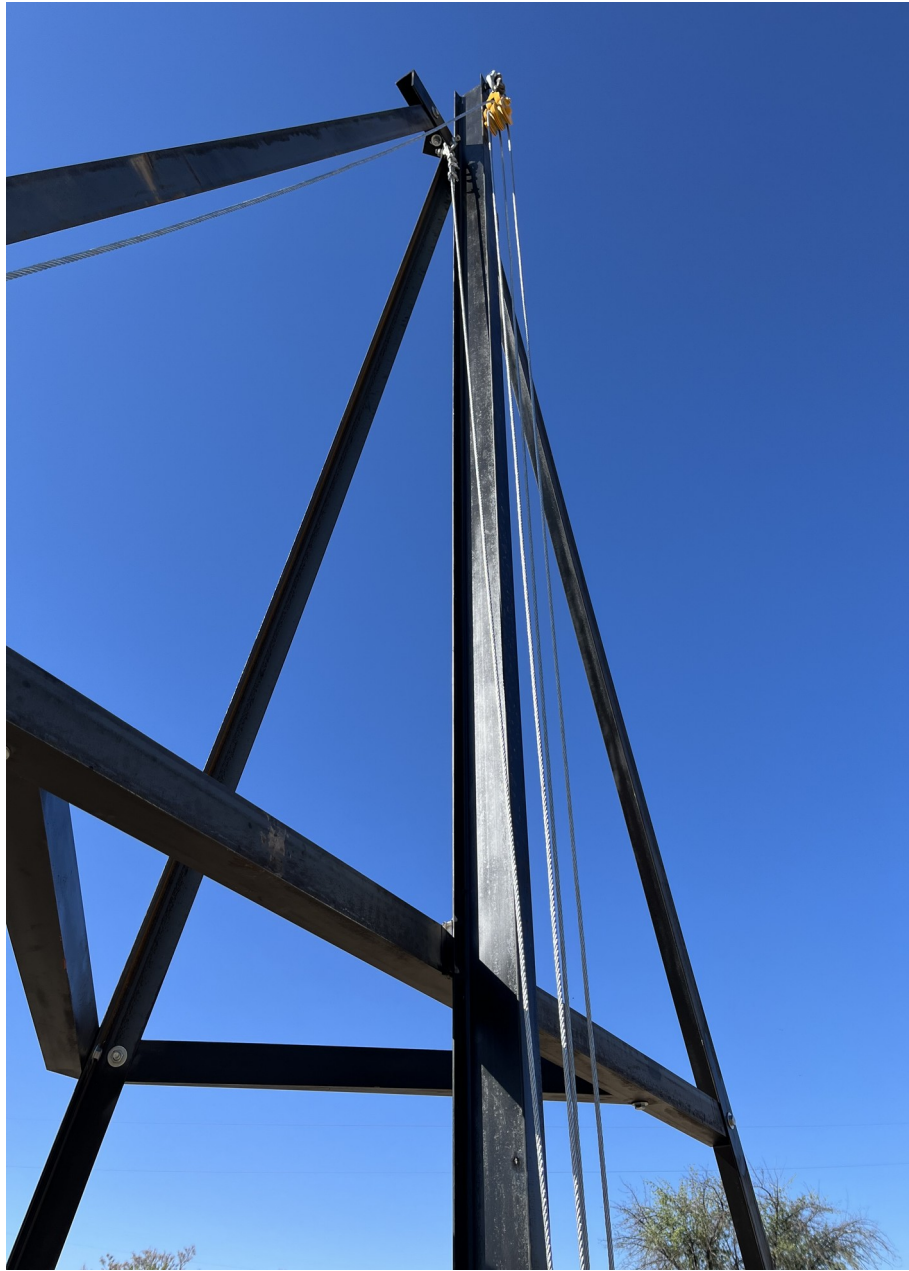
Figure 31. Upper end of the pulley lift (5MAY2023).
