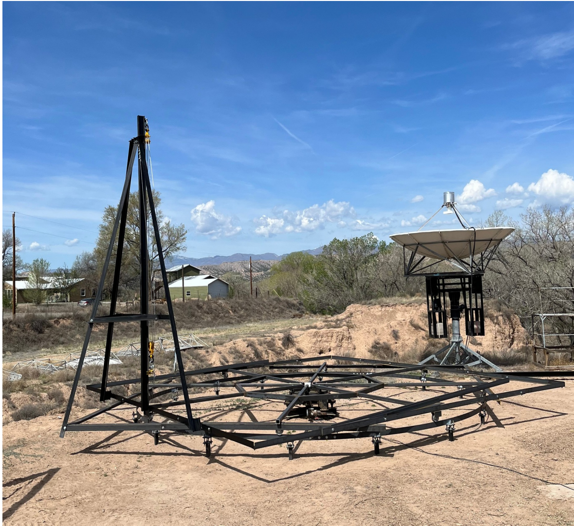
Figure 30. First lift tripod is shown installed on the AZ mount rotating base structure (3MAY2023).
