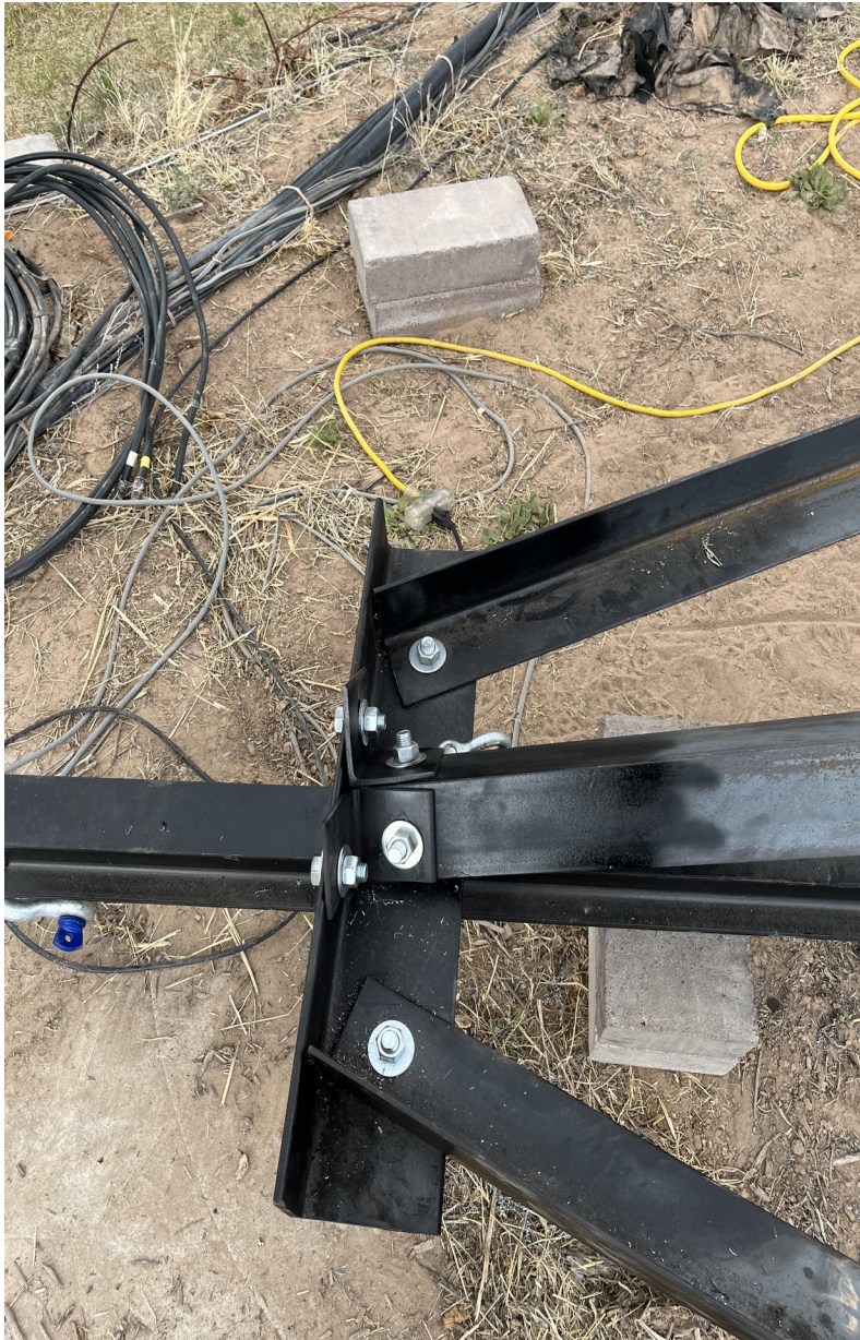
Figure 23. Upper end beam attachment configurations.
