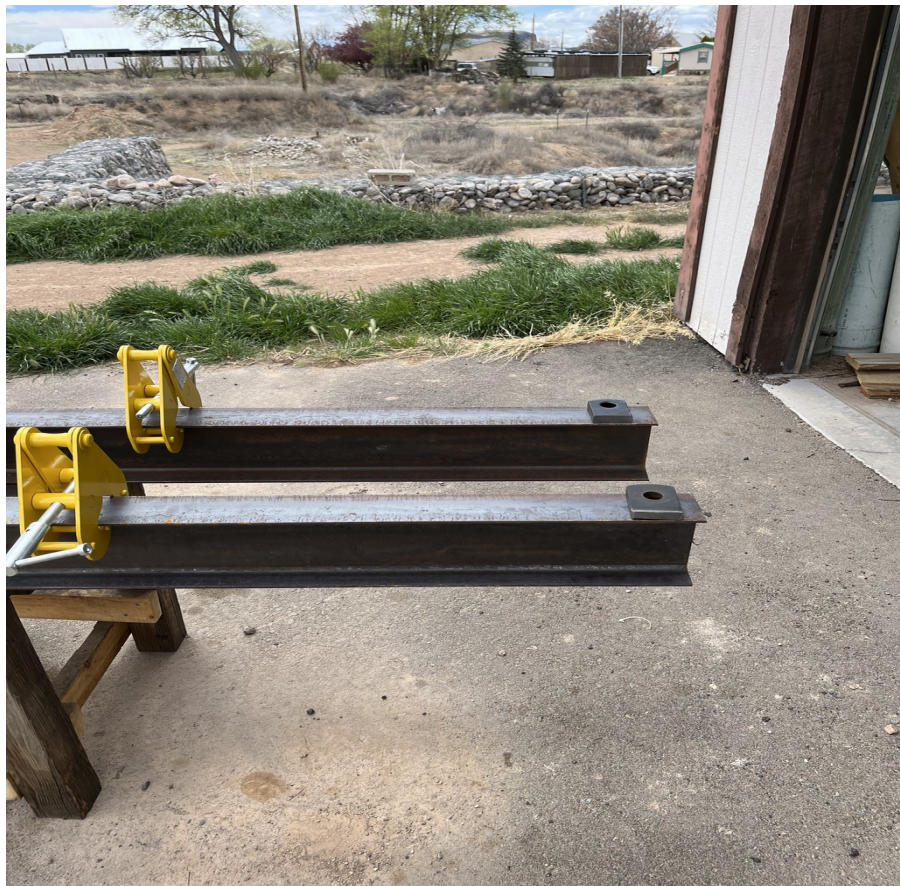
Figure 10. Two steel tabs that will become lifting brackets are shown above.
