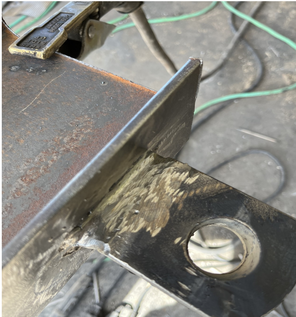
Figure 14. Root weld for the lifting tab is shown above (27APR2023).
