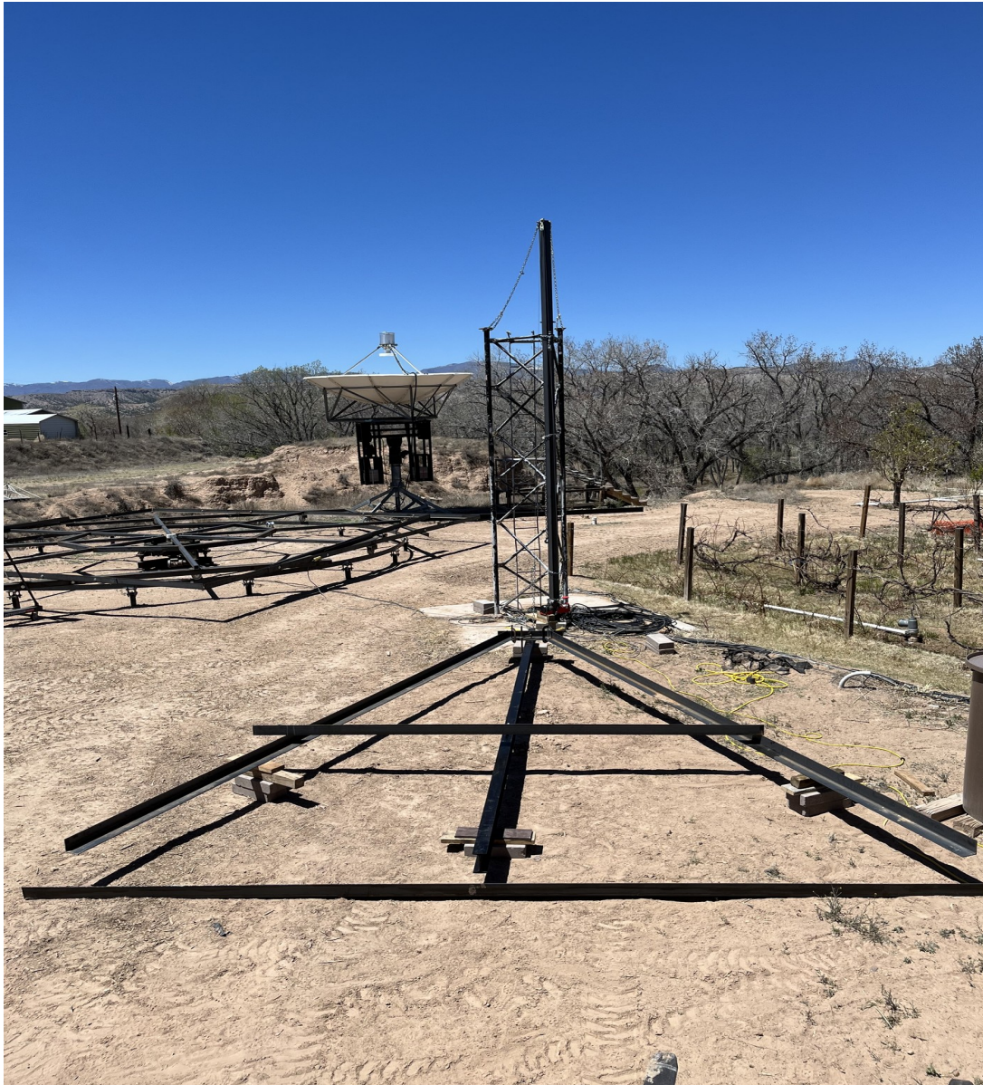
Figure 17. Principal side of the first lift tripod under construction (29APR2023).
