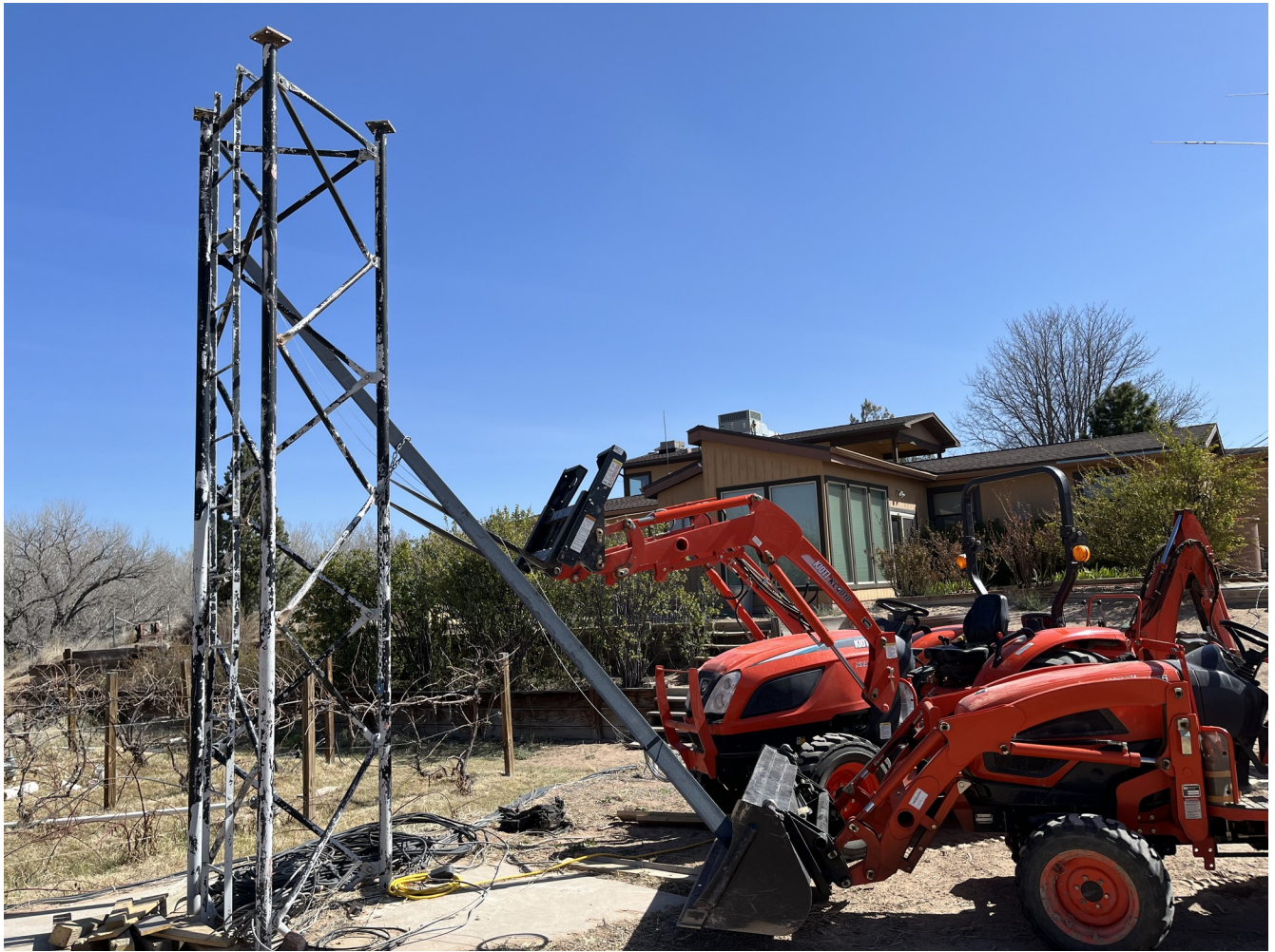
Figure 7. Positioning the pre-rigged temporary lift beam using two tractors.
