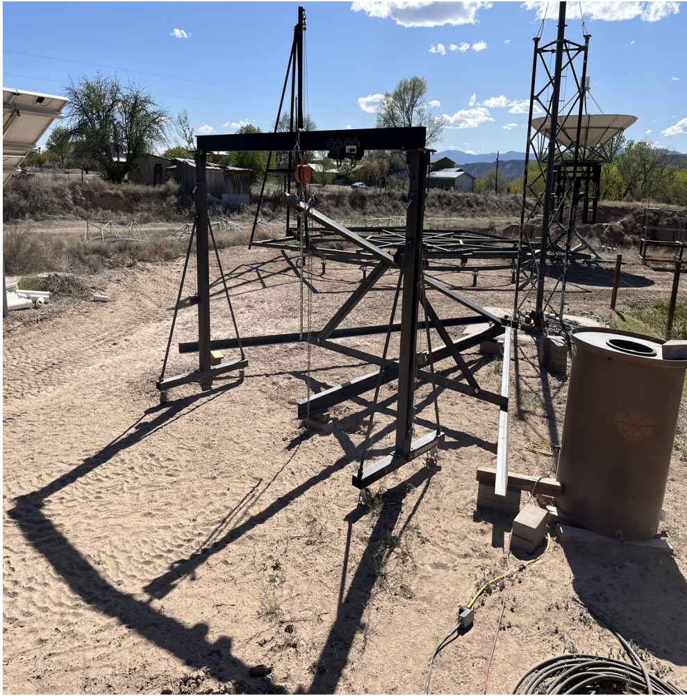
Figure 33. Fabrication of the second lift tripod is nearly completed (6MAY2023).
