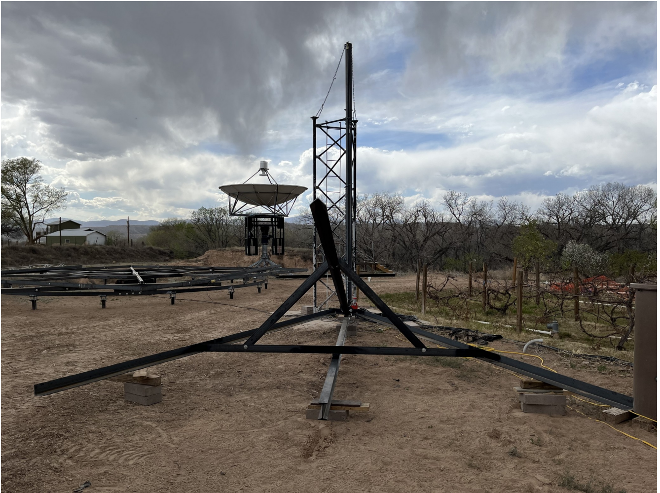
Figure 24. First tripod structure fabrication is shown completed (1MAY2023).
