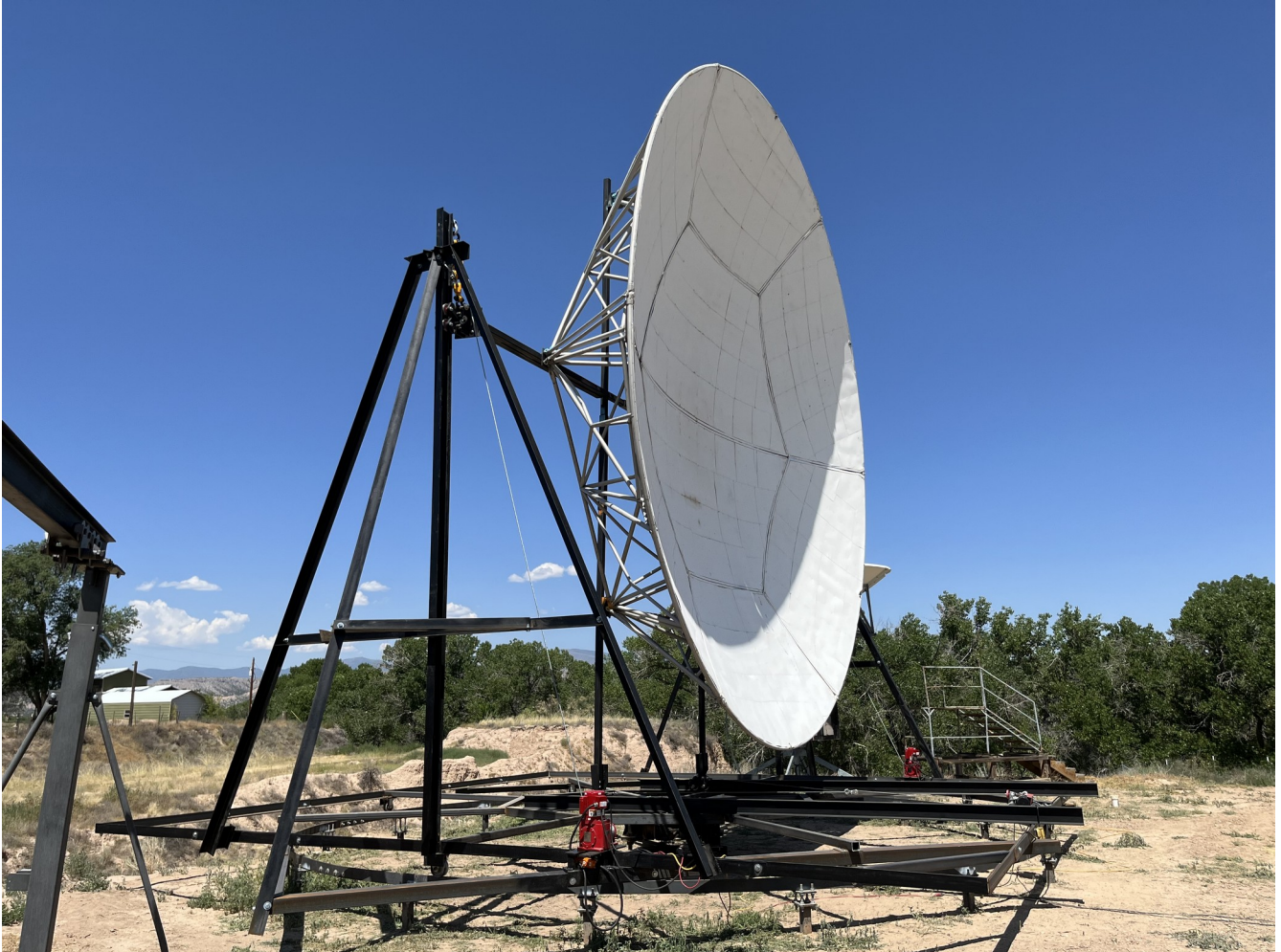
Figure 5. Dish shown at zero degrees elevation angle in maintenance mode (25JUL2023).
