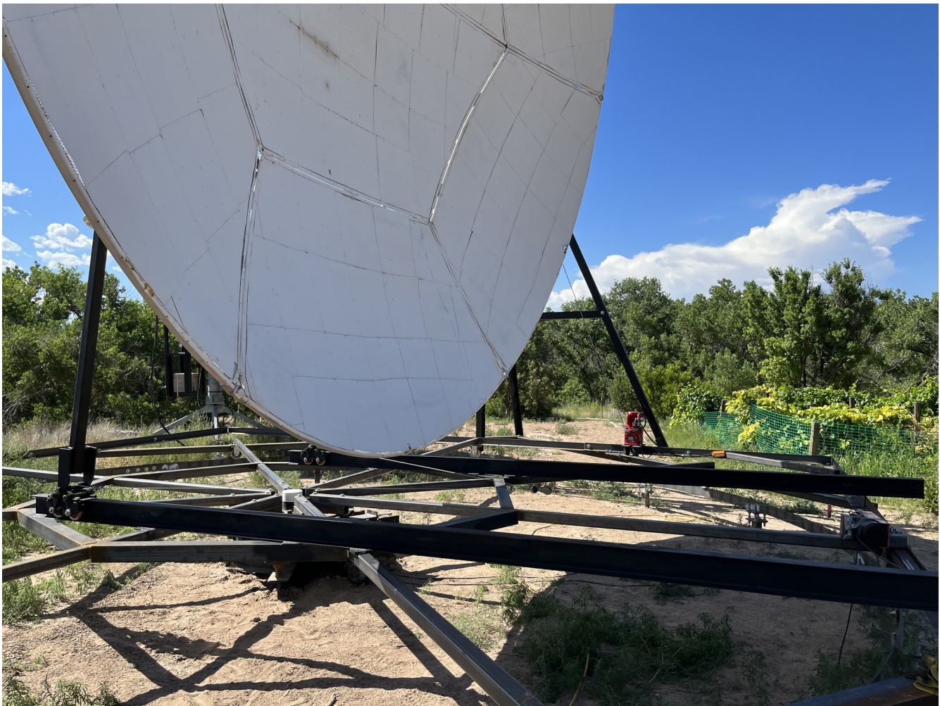
Figure 3. Configuration after the trolleys have been re-established onto the I-beams (23JUL2023).
