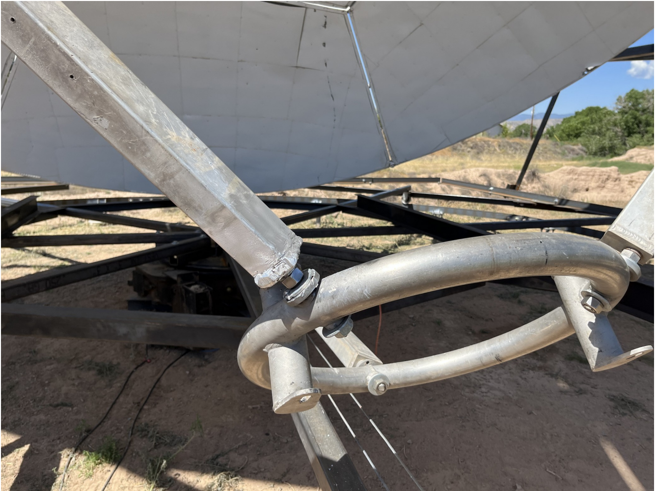
Figure 18. View showing the completed aluminum weld of the support beam.
