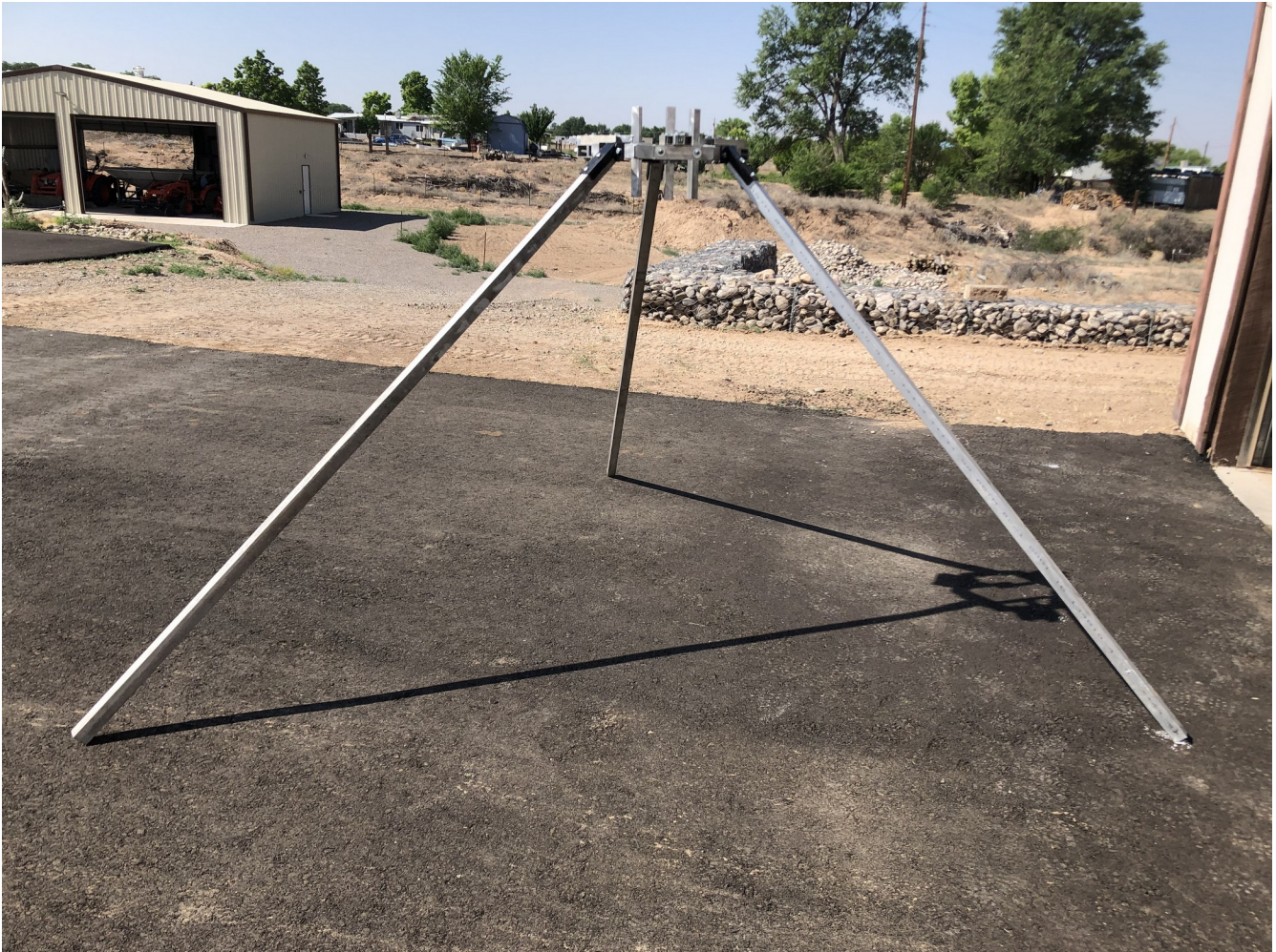
Figure IV-38. The feed support arms are bolted onto the hexagon mounting ring.
