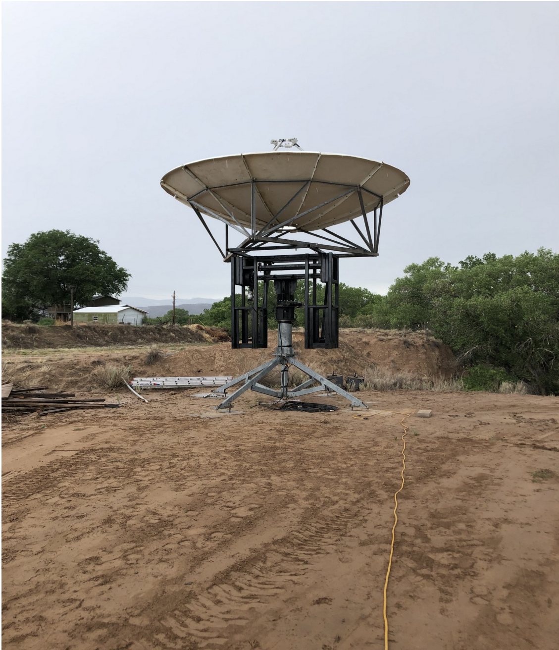
Figure IV-62. Dish installation completed as rain began falling. Timing was fortuitous.
