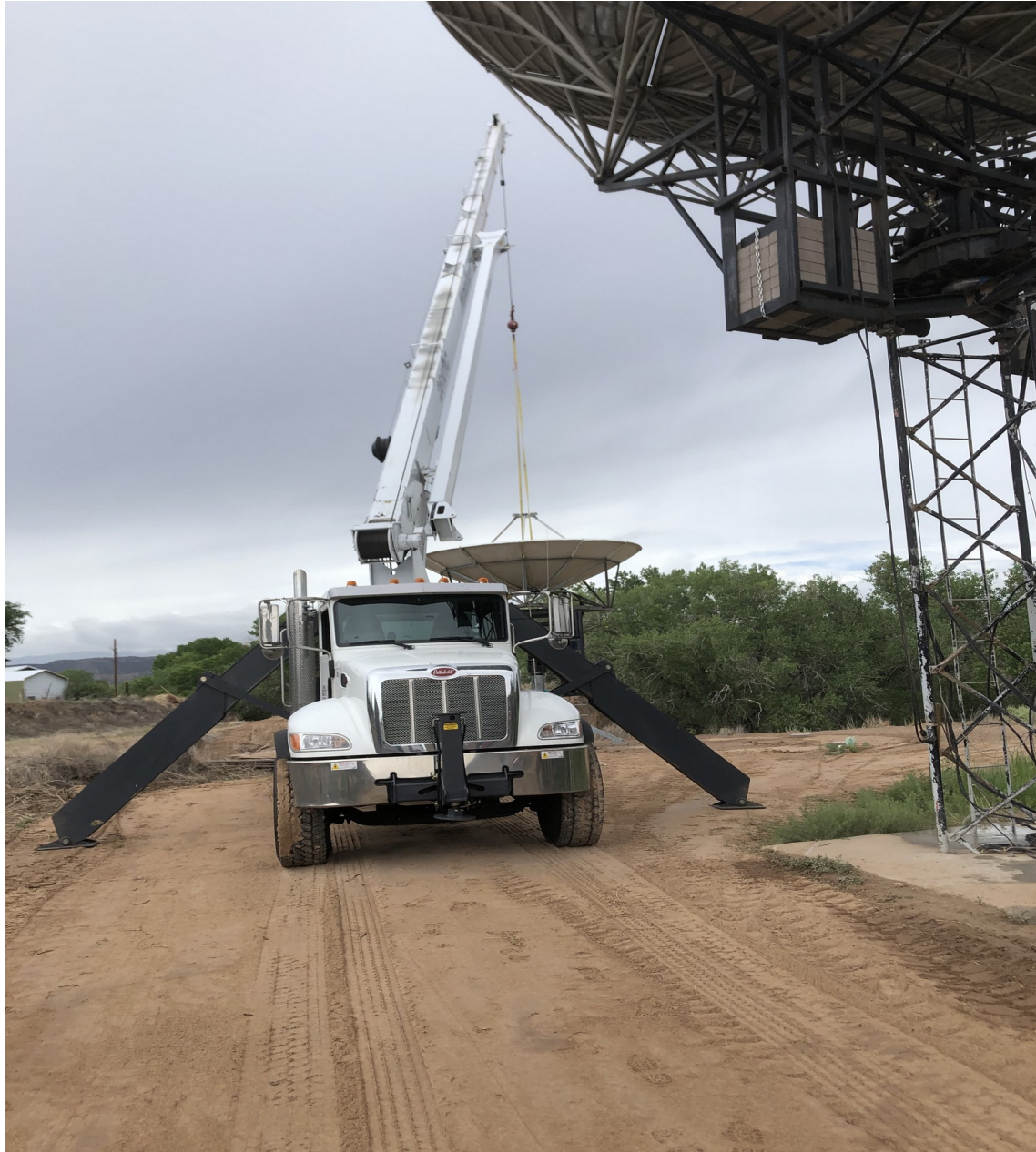
Figure IV-60. The dish is being set atop the AZ/EL mount by the crane.
