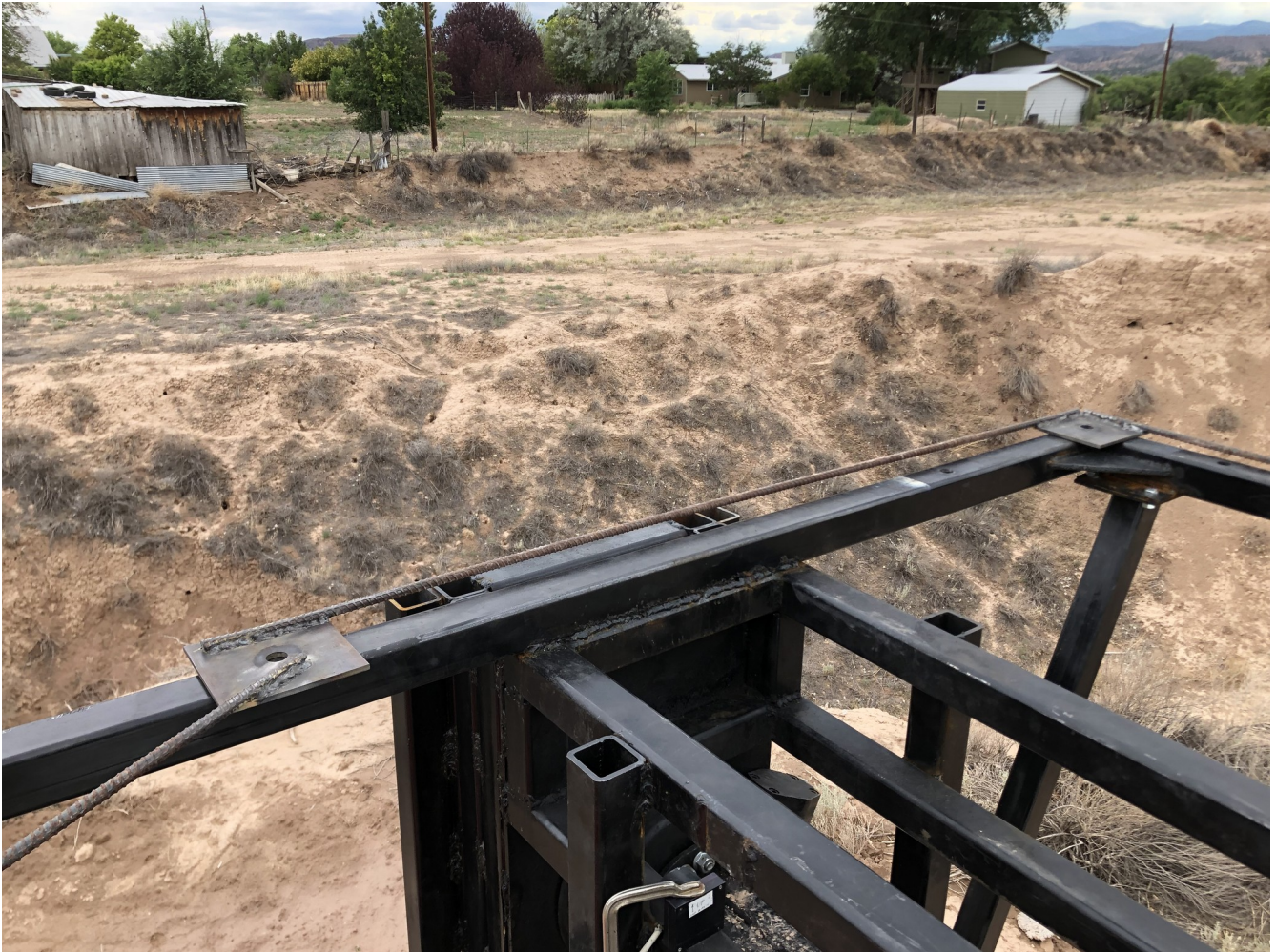
Figure IV-54. Two plates of the rigid template in position after rotating the completed template 180 degrees.
