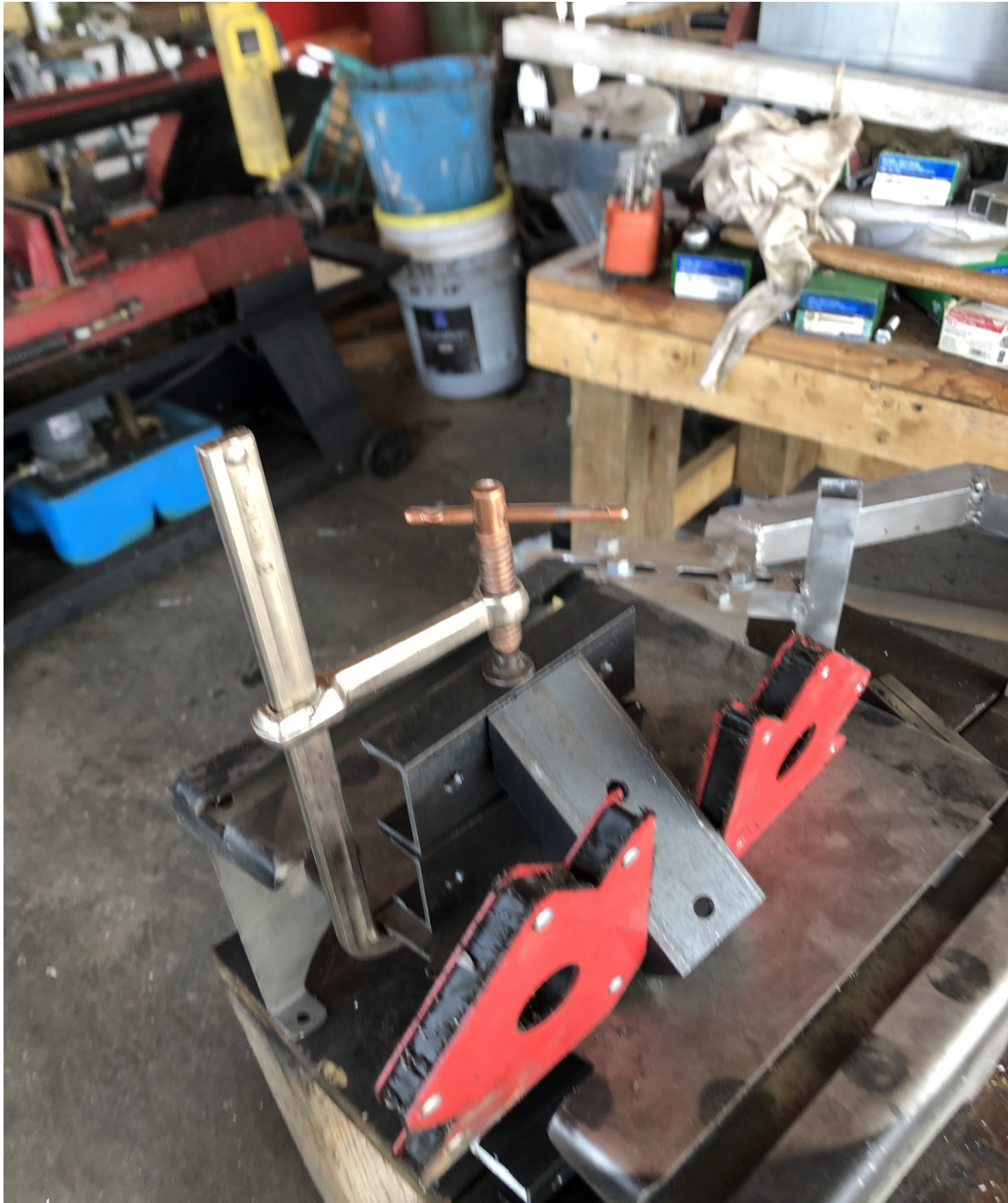
Figure IV-33. An upper end bracket drilled and clamped for welding. Note the use of two welding magnets used to keep the angled piece in place during welding.
