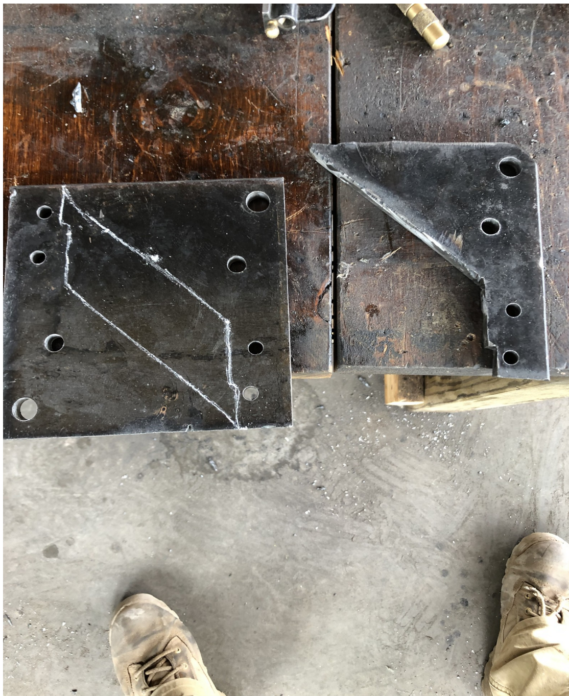
Figure IV-42. Plate (left) drilled and marked prior to cutting the bracket elements. A cut and drilled bracket element is also shown (right).
