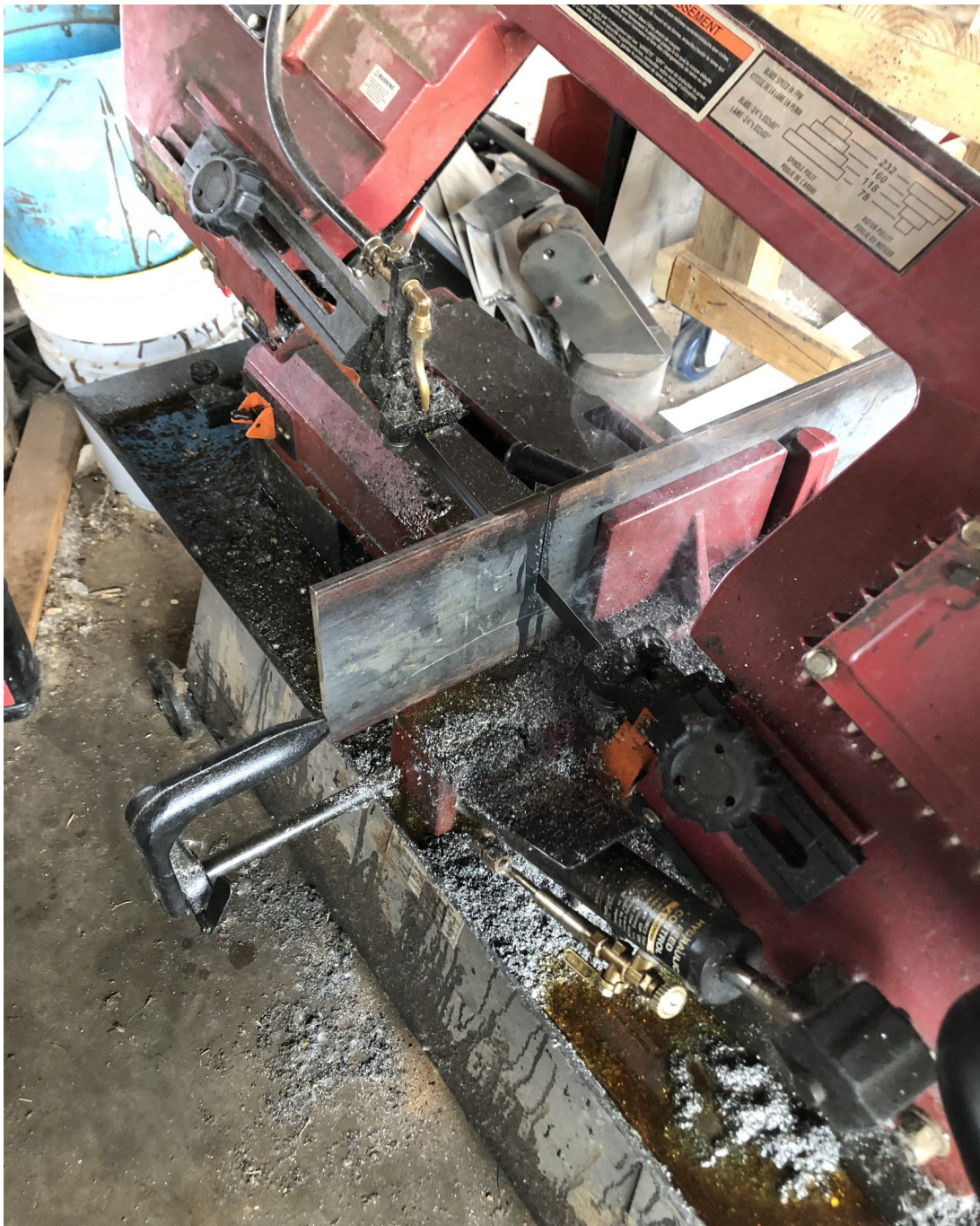
Figure IV-48. Cutting six 6" square bolt plates that will form the rigid drilling template.
