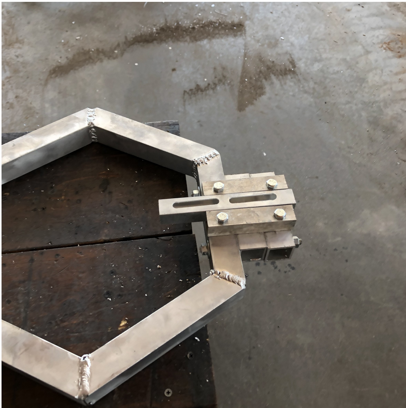
Figure IV-27. Two guides for the slotted support for this hexagon side are bolted into place using through 3" long 3/8"-16 bolts with nuts on the underside.
