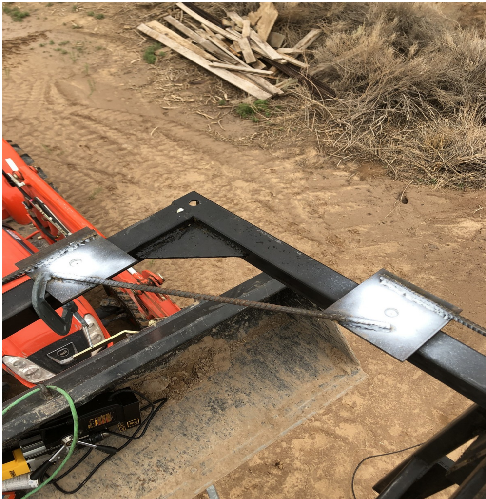
IV-56. New hole positions marked with white paint and center punched.
