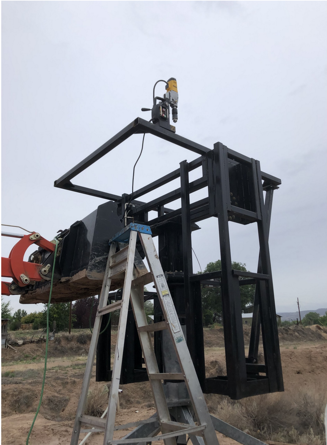
Figure IV-57. A magnetic drill press in position to drill new through holes.
