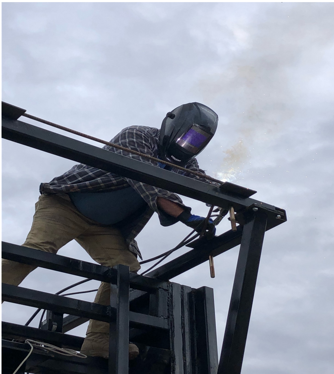
Figure IV-52. Rebar connecting rods being welded onto the template plates.
