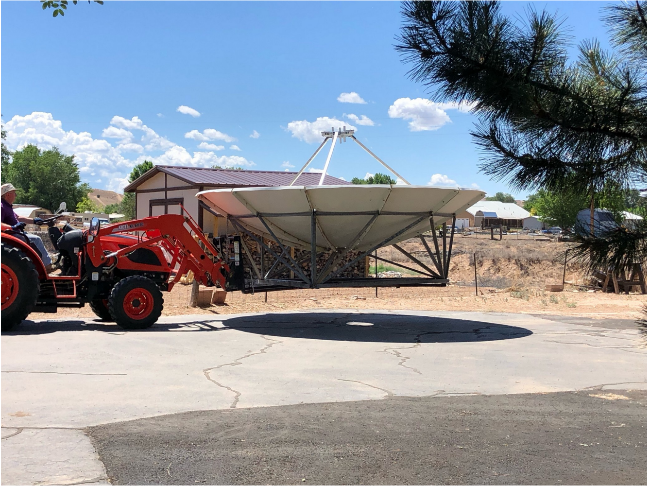
Figure IV-46. 4.6m dish being moved to the AZ/EL mount location.
