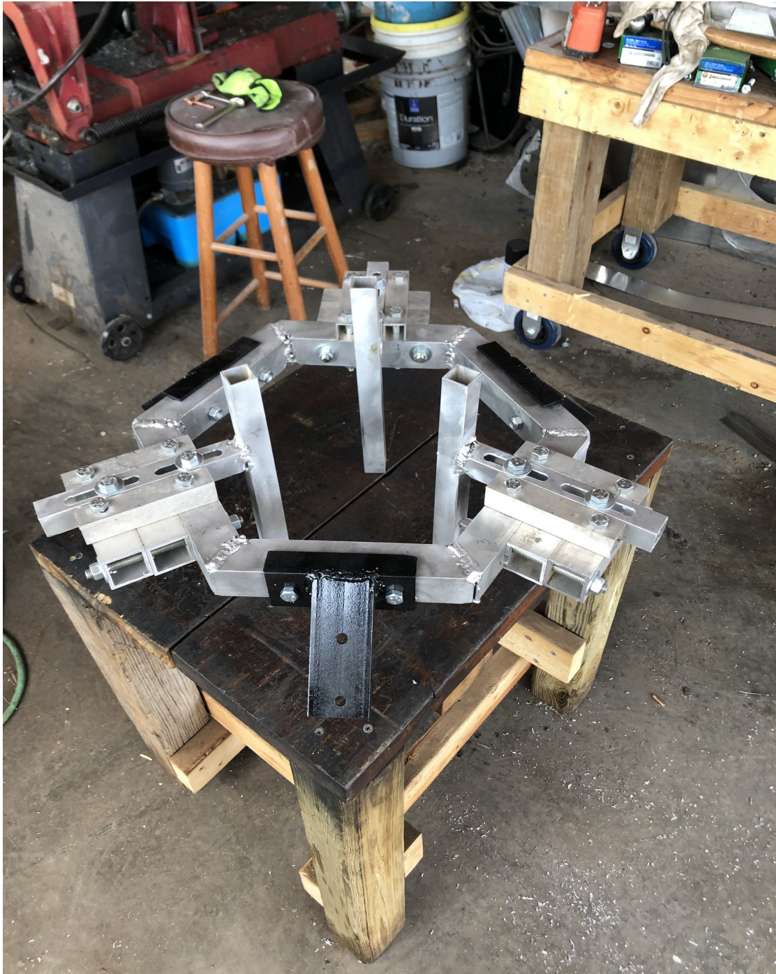
Figure IV-35. Upper end feed horn strut brackets are completed and installed on the hexagon feed horn support ring. The upper end of the feed horn support structure is now complete.
